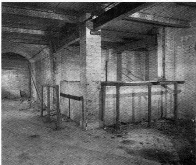
Servery in the Ashley Road deep shelter in Epsom, Surrey. Photo by Nick Catford
